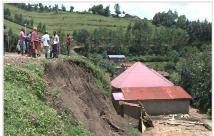
Nyabihu: Houses get destroyed by landslides due to roads missing water drainage.
