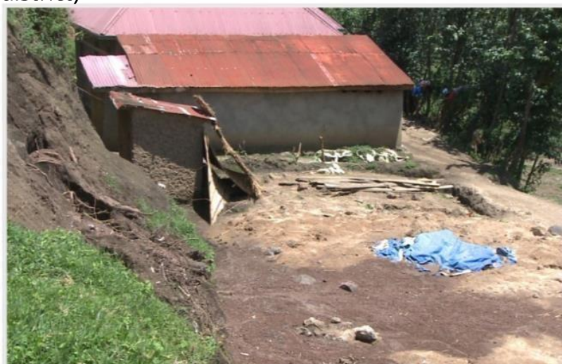
Nyabihu: Houses get destroyed by landslides due to roads missing water drainage.
